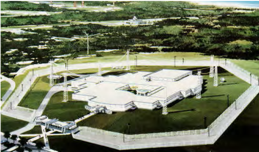
Figure 4.4-1 Morrell Operations Center (MOC), CCAFS
